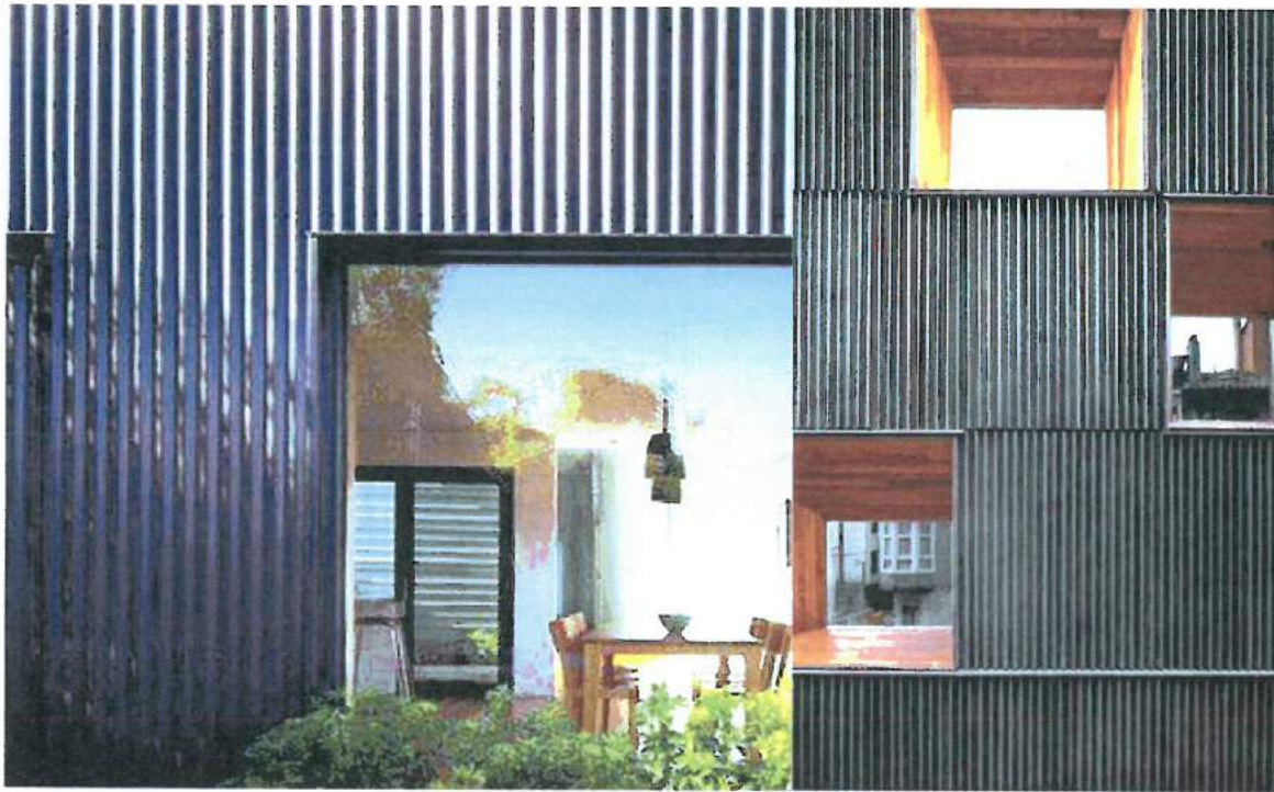
Vertical Profiled Metal Panel
