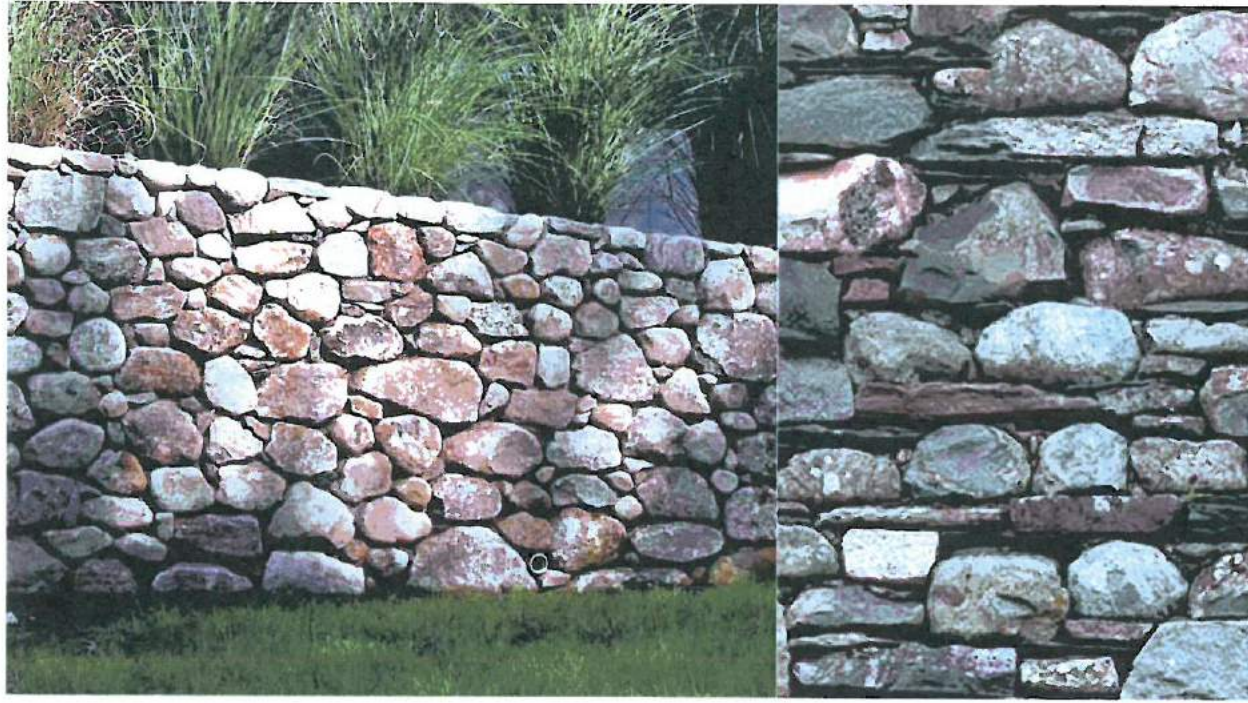
Rubble Stone Retaining Wall
