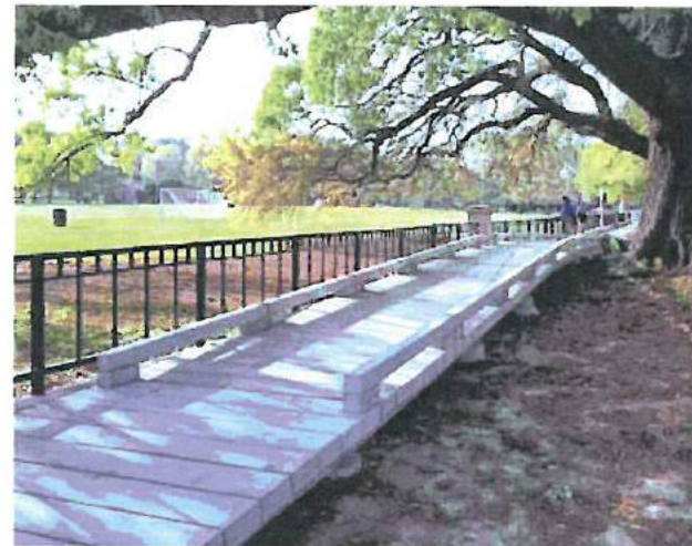
Raised wood or metal path adjacent to heritage trees
