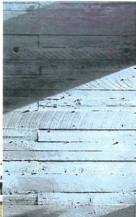
Board Formed Concrete
